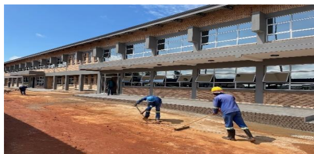
Construction of HMIS/BioMed Offices at 97% completion
